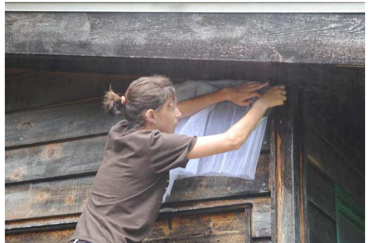
Applying screen for one-way door
